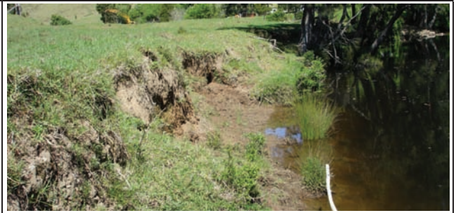
Minor to moderate active erosion: exposed tree roots
