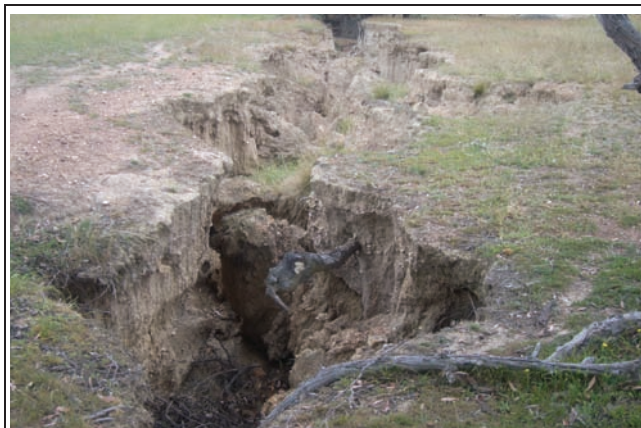
Very high to high risk: significant active erosion and headcutting
